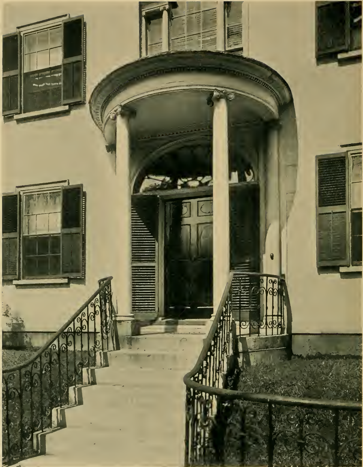
DETAIL OF ENTRANCE PORCH AND DOORWAY, LANGLEY BOARDMAN HOUSE, PORTSMOUTH, NEW HAMPSHIRE.
